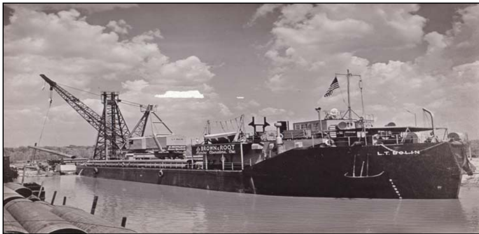
Figure 5.14. Brown and Root Pipe Laying Barge. Photo Courtesy of Jesse Grice Collection, Morgan City Archives.
