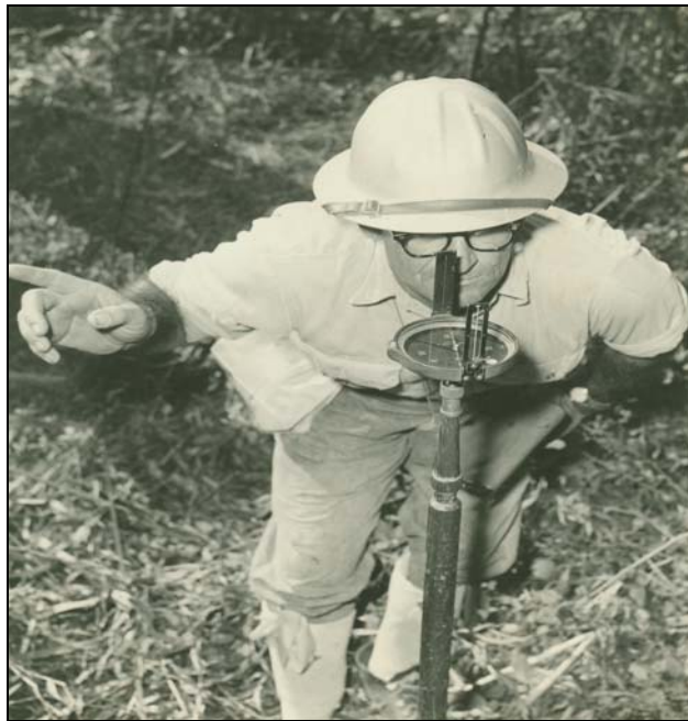
Figure 4.1. Nelson Constant Using Breton Compass While Surveying in the Marsh. Photo Courtesy of Nelson Constant, OOGHP.
