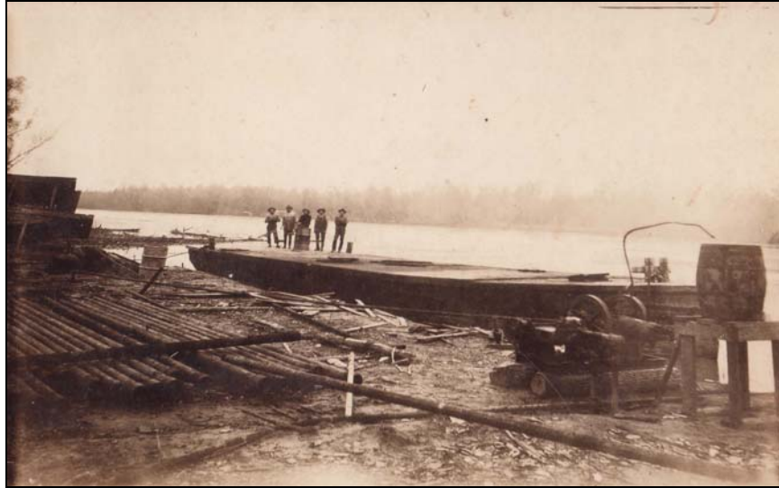
Figure 3.6. A Crew Loading Pipe onto a Barge on the Atchafalaya River, to be Floated to a Texaco Rig, 1924. Photo Courtesy of Doughty Dominique, OOGHP.
