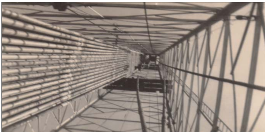
Figure 5.15. Looking Straight Up a Derrick, Drill Pipes Stacked Against One Side. Photo Courtesy of James Broussard, OOGHP.
